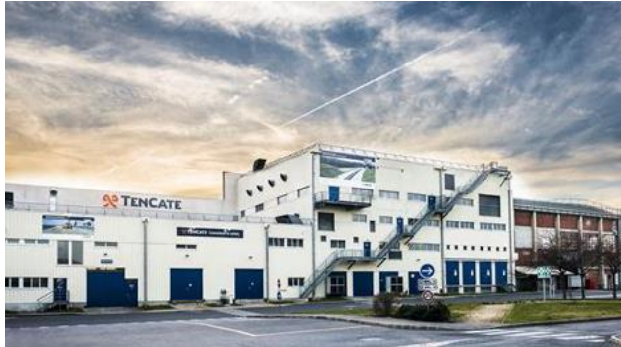
TenCate Geosynthetics Plant in Bezons, France
